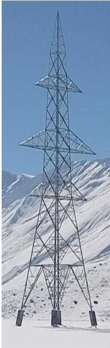
Raised Chimney Foundation (for snow deposit area)
